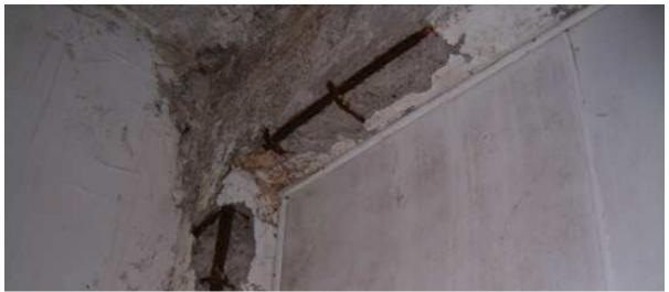
Corner showing rusting structural steel and water damage
