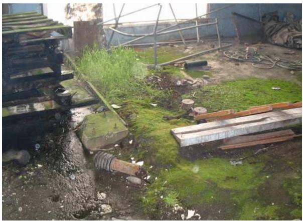
Water damage inside building from leaking internal gutters.
