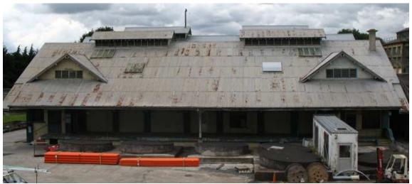
This photograph shows the roof in need of repair. It also has the concrete plinths in the front and the access way (white building) added later, which we would like to remove
