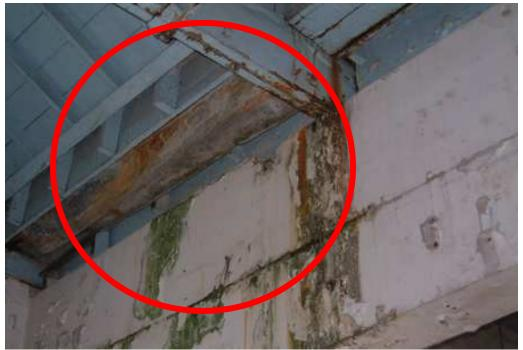
Internal gutter has been replaced with tin which has collapsed.
