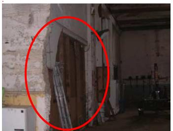
Hole cut in wall adjacent to hole with structural column hanging down.
