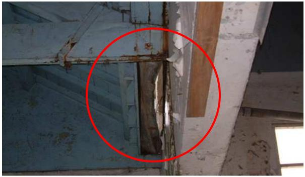
Collapsed tin gutter.
