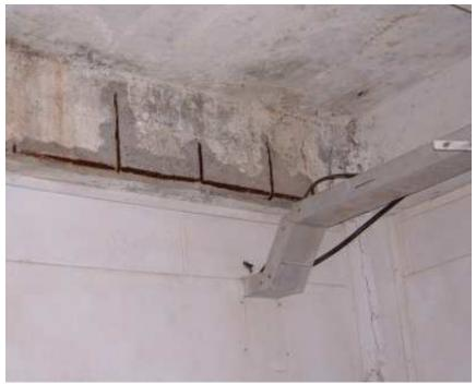
Shot of roof showing rusted structural steel
