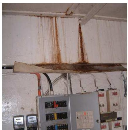
Water damage through roof and onto switch gear.
