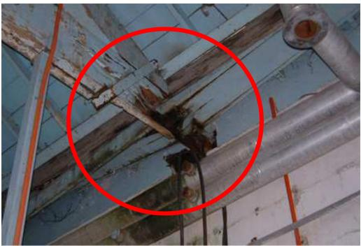
Leaking internal gutter, rotting trusses.
