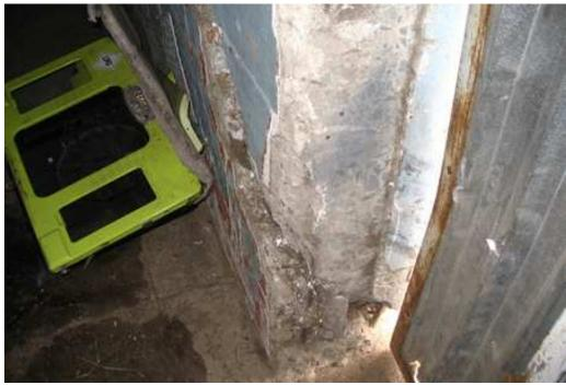
Damage to the back wall where the front end loader has been driven into the structural column.
