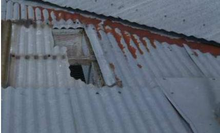
Broken clear corrugated panel needs to be replaced and resealed.
