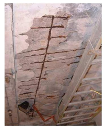
Structural steel rusting and blowing concrete.
