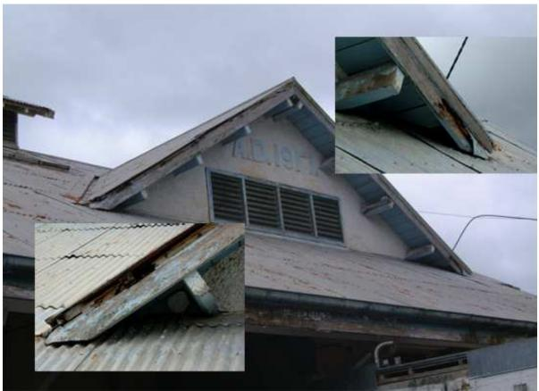
Fascia and barge boards are rotting and need to be replaced
