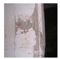
Damage to the other side of the wall including holes in the wall and damage to the structural column beside the removed column.
