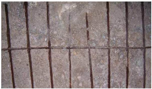
Shot of roof showing rusted structural steel
