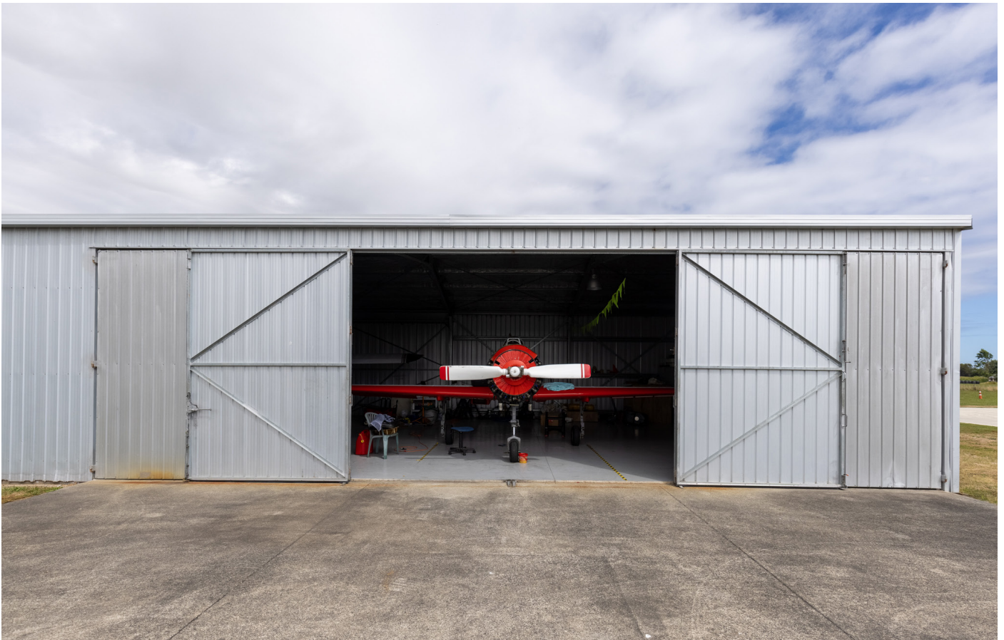
Photo 12. An example of how the hangars are constructed to accommodate aircraft with large double folding doors. This particular plane is another Russian Yak that regularly participates in Waka Warbirds.
