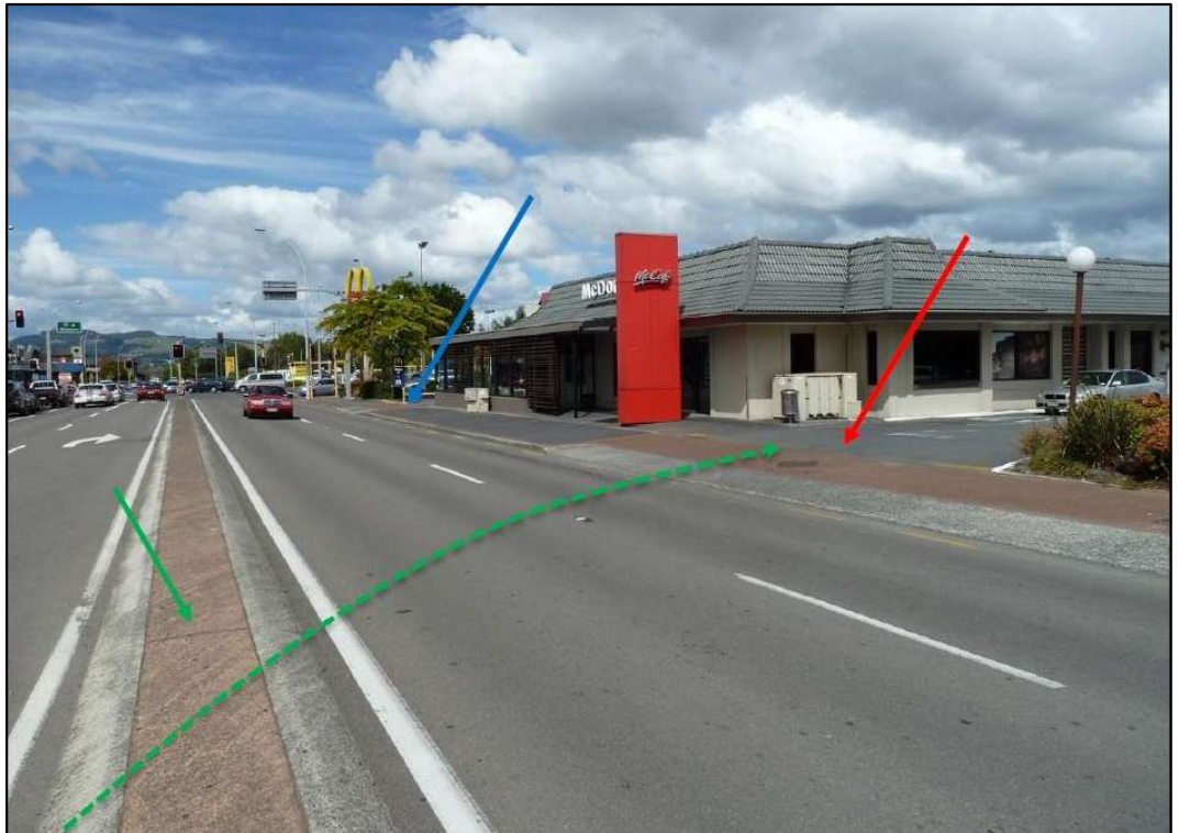
Figure 5: SH30A exit from McDonald's Rotorua (red arrow), with SH30A entry (blue arrow), and tyre marks across central median (green arrow). The green dashed line illustrates the assumed path of a road user
