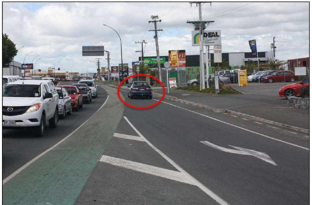
Figure 4: Right turn out exit from Burger King Te Rapa (Hamilton) into opposing left turn slip lane (vehicle circled) for northbound left turn from Te Rapa Road onto Wairere Drive
