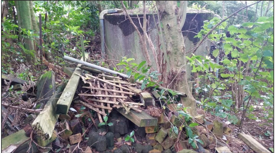
Photo G: Water tank and retained “cut” into bank (retains driveway above).
