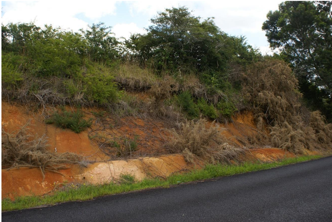
Plate 2: Weavers Crossing embankment of ~ 5 m height and ~ 30° slope-angle
