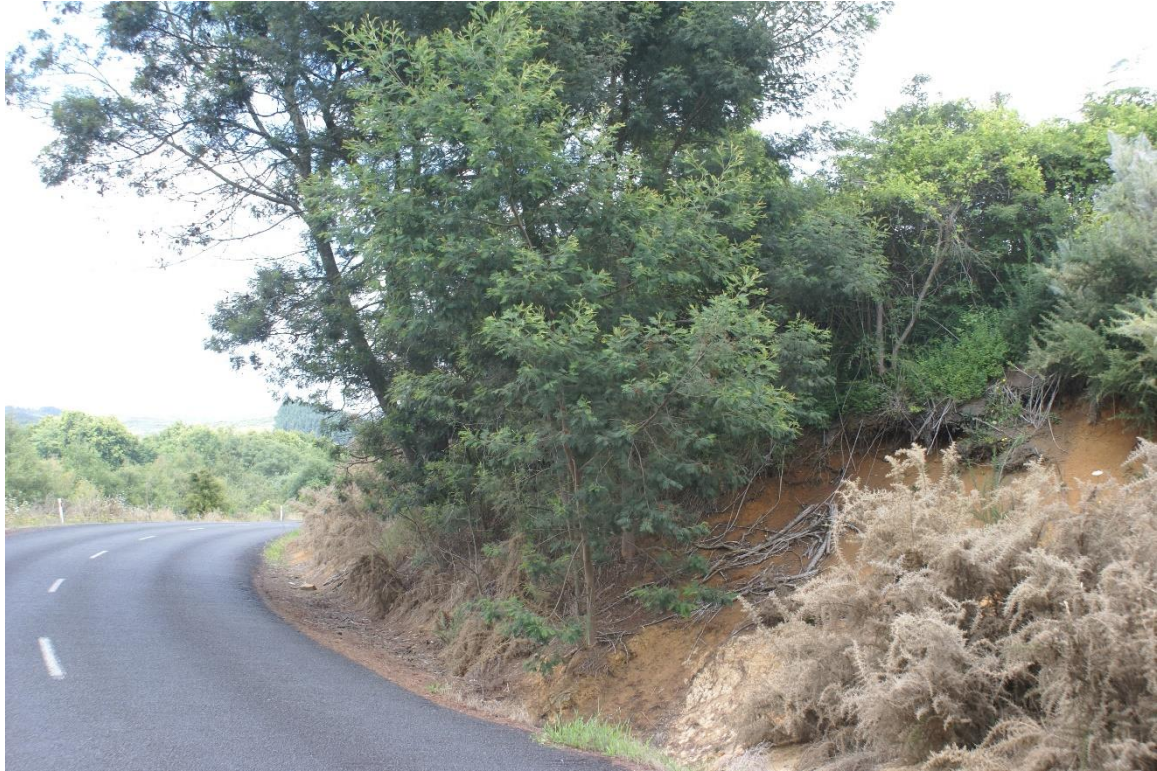
Plate 5: Leaning trees on the road embankment indicating some shallow down-slope displacement near the bottom of the slope
