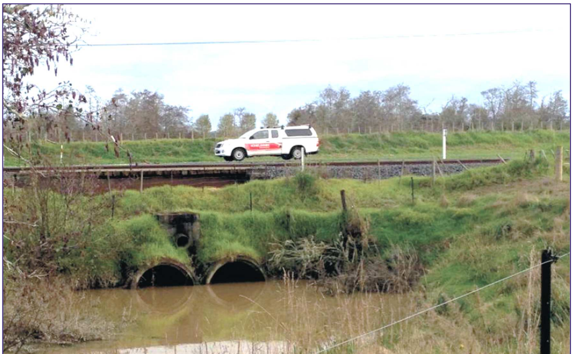
Figure 2.2 Flood-gated culvert outfall of Kimihia stream into Waikato River.
