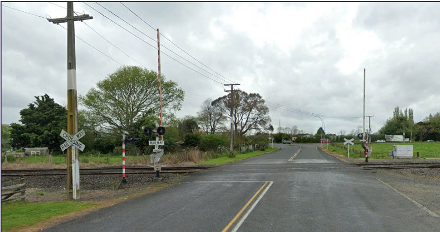
Figure No. 5: NIMT Level Crossing on East Mine Road
