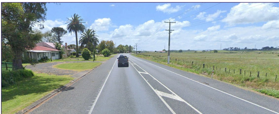
Figure No. 4: State Highway 1/ Great South Road looking north (Source: Google Street View)
