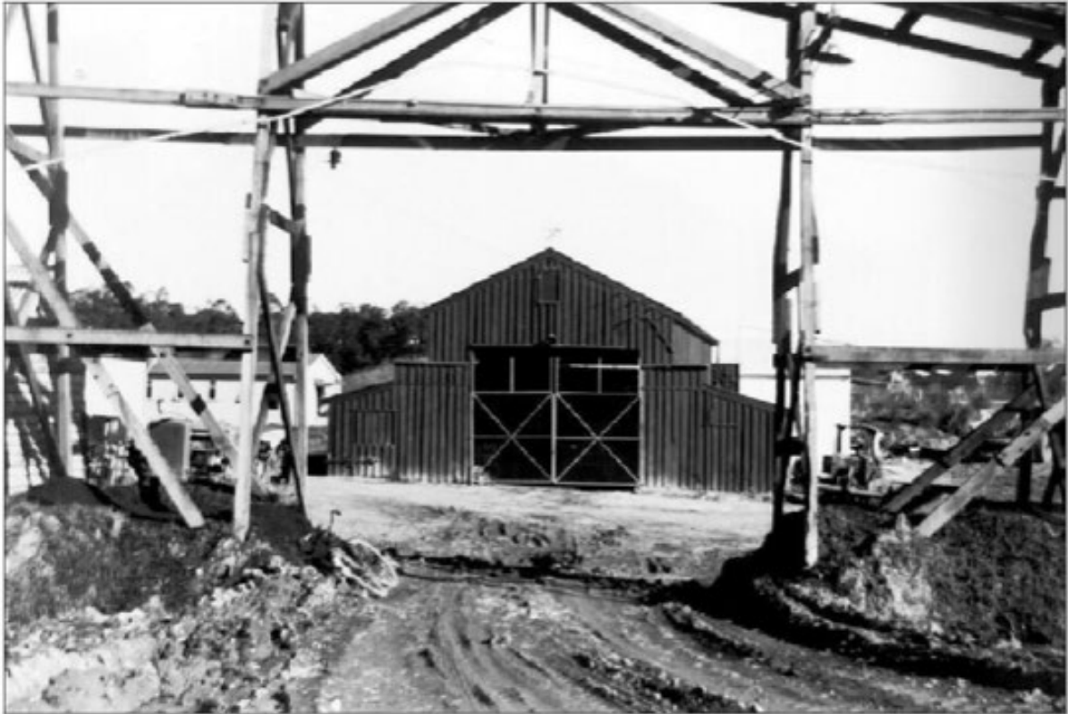
The main workshop viewed through the trestle supports for the conveyor belt which brought the coal up from the pit.
