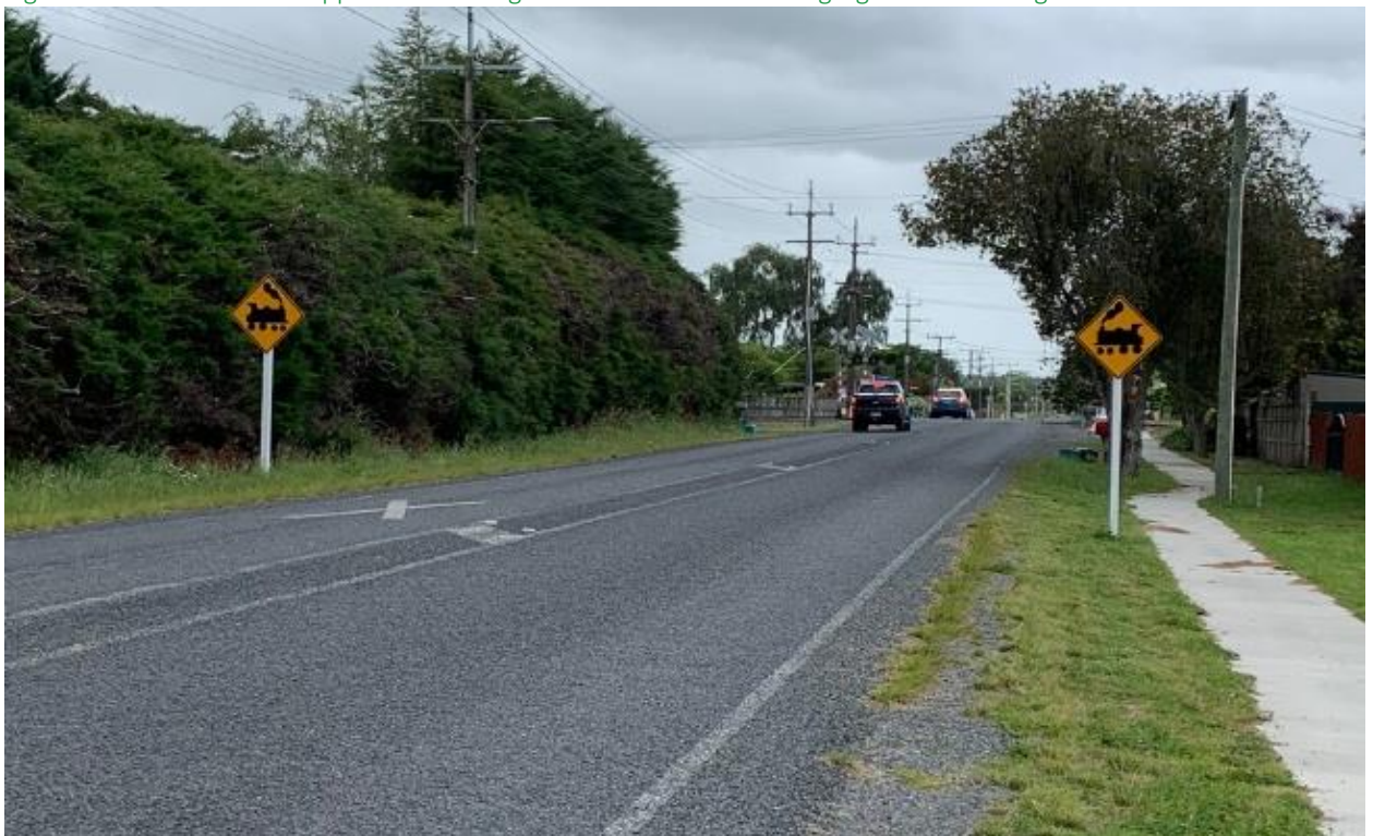
Figure 9: View on eastern approach showing correct advanced warning signs and markings
