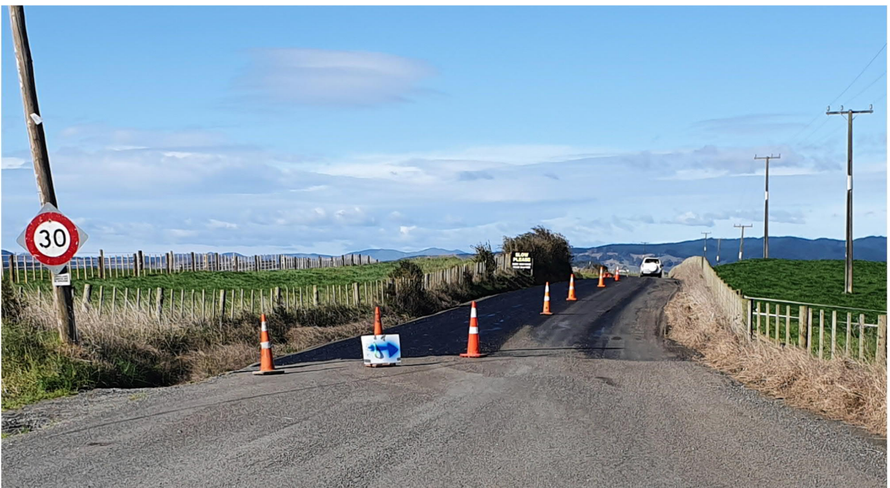
Figure 5: Murray Christensen Road as of July 2020 (sealing of carriageway)
