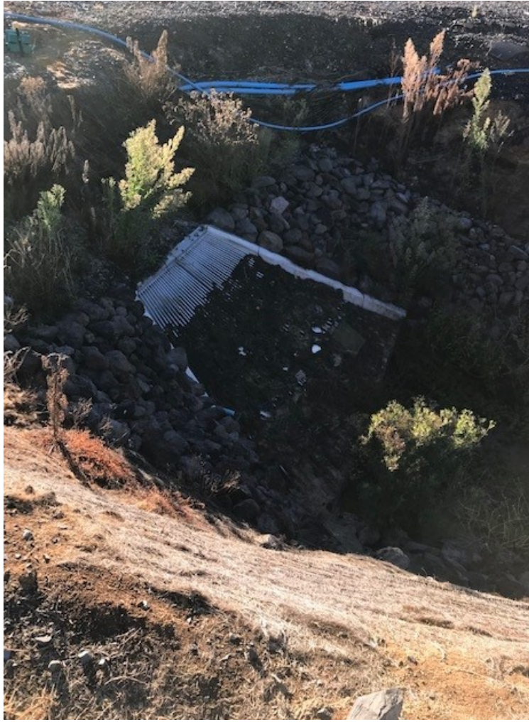
Inlet under entrance to the Synlait site (end of ditch along McDonald Road west of roundabout)
