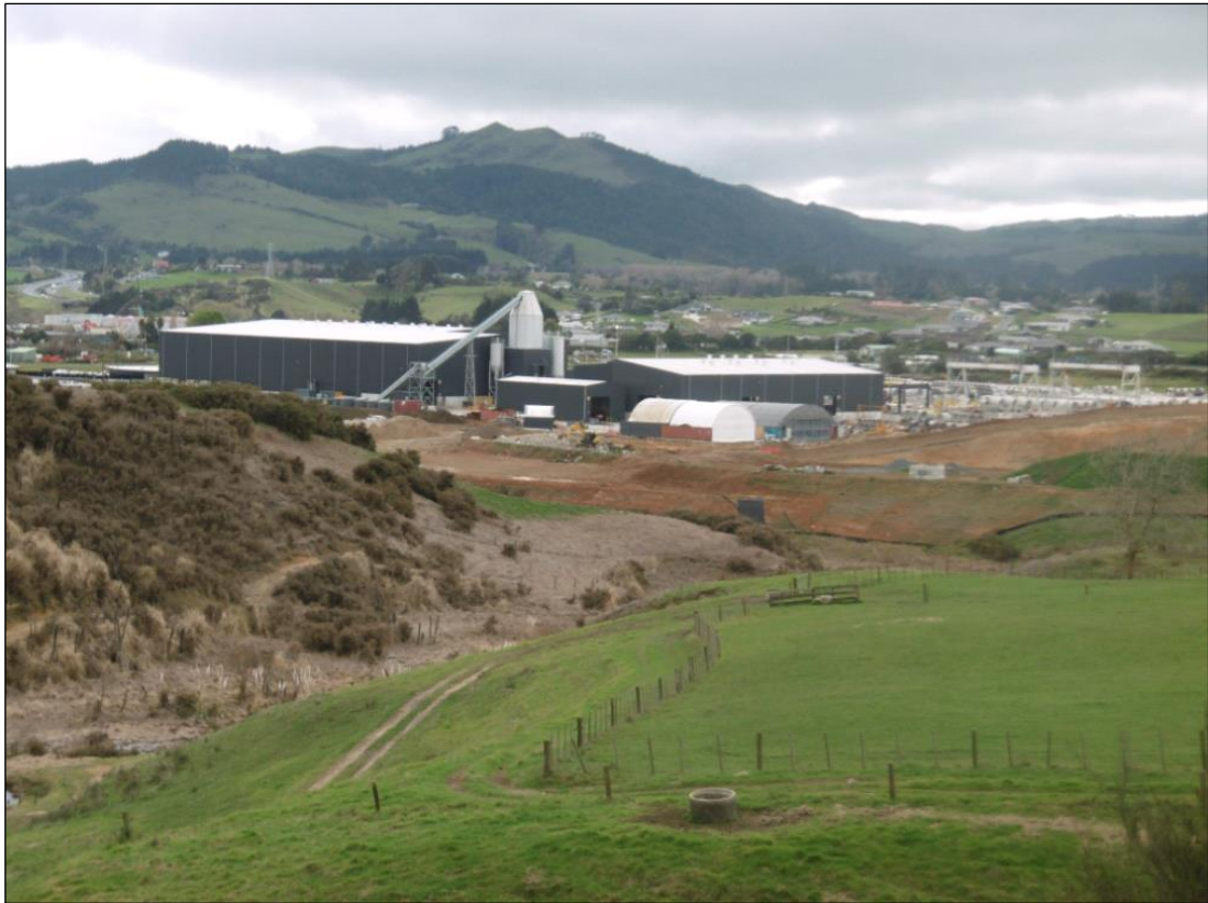
Figure 4 Photo showing batching plant (16m) and batching tower (29m). Photo is taken from 62 Bluff Road site.
