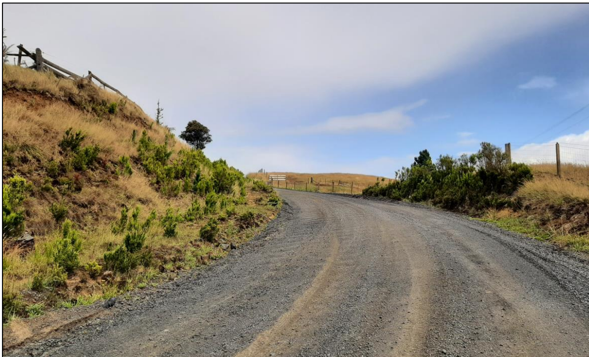
Figure 4: Signs of Benching
