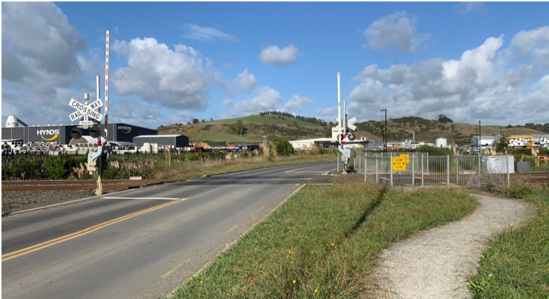
Photograph 2: McDonald Road rail crossing
