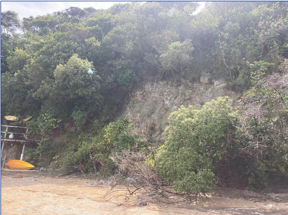
Figure 49: Shoreline in Section 2 (fronting 2c Ryan Road). Note evidence of recent slope failure (slip occurred in 2020).
