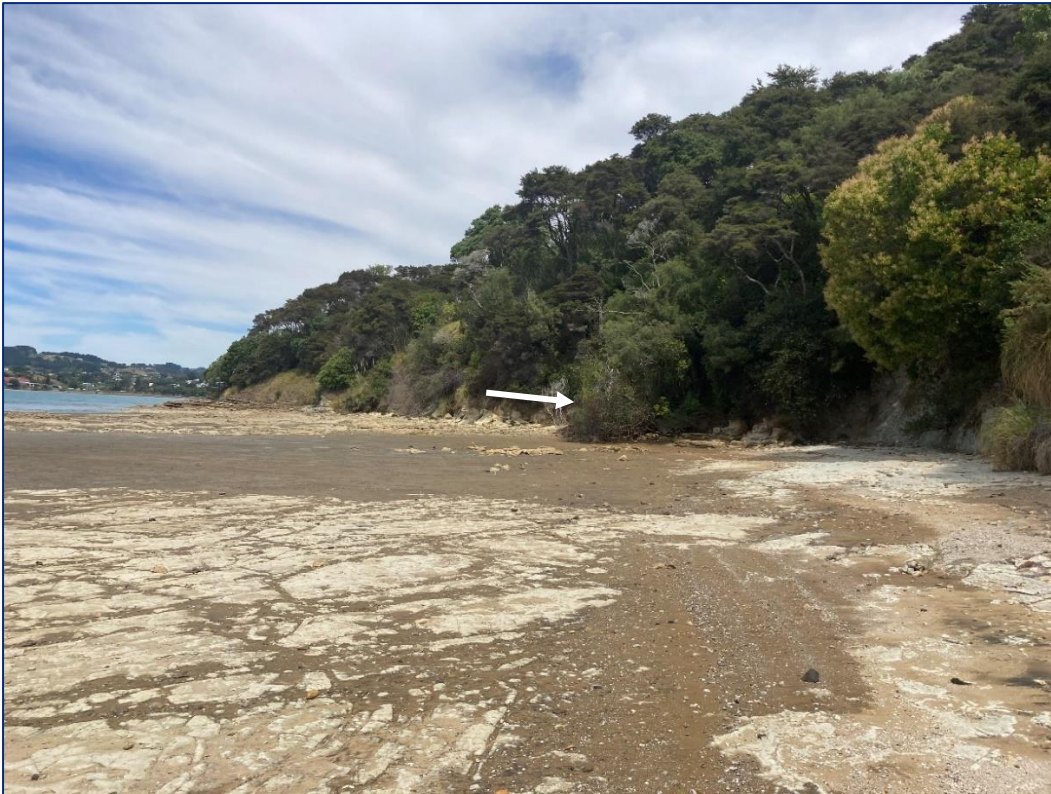
Figure 53: Eastern Shoreline. Approximate location of recent land slip indicated by white arrow.
