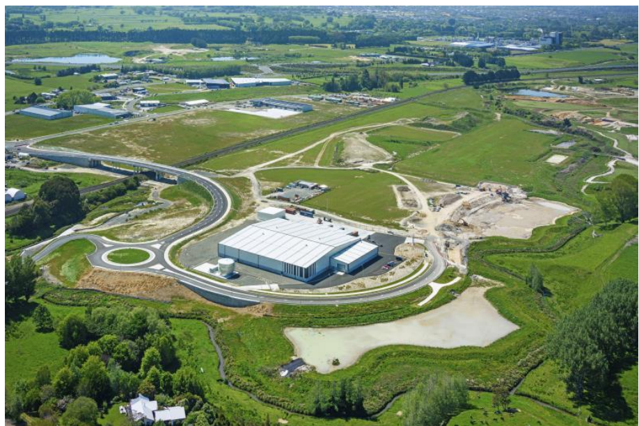
Figure 2: Waikato Freight Hub development as at November 2019
