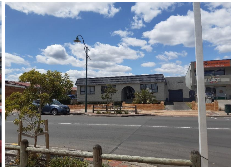
Empty office space (for sale) on George Street.
