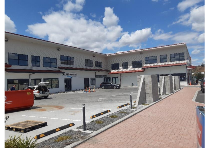
Building under construction on Great South Road.
