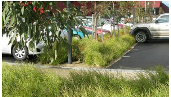
Figure 15. Precedent Image: Use of rain gardens and other low impact design techniques within car parks will reduce stormwater runoff.
