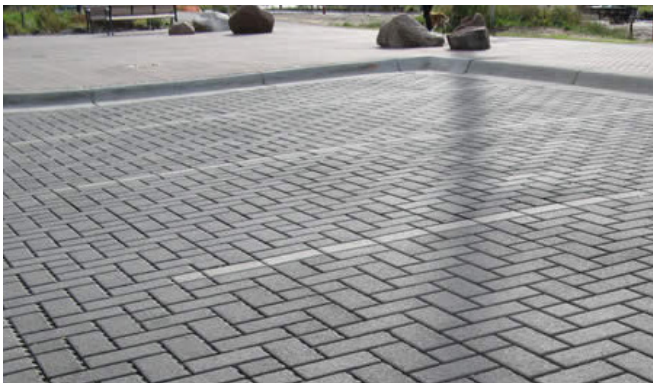
Figure 14. Precedent Image: Use of porous pavement materials within car parks will reduce stormwater runoff.
