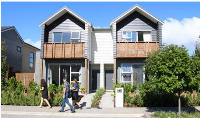
Figure 7. Precedent Image: Clearly visible front entrance.
