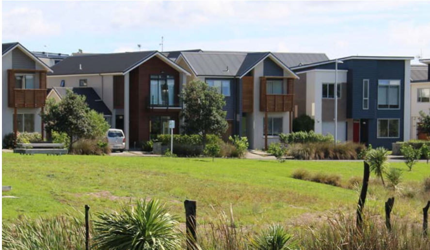
Figure 5. Precedent Image: Consistent building form, including heights and architectural styles, adds positively to amenity and character.
