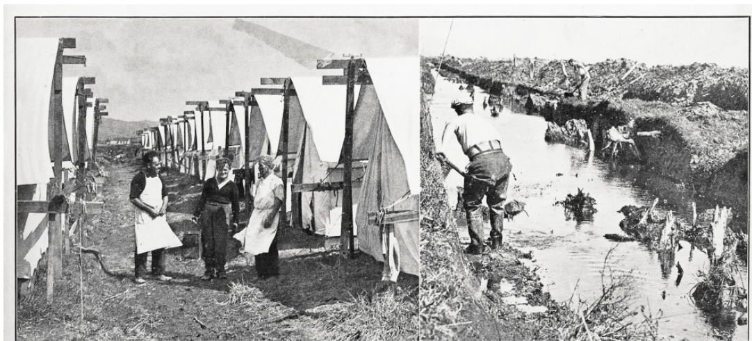
USEFUL DRAINAGE WORK BEING CARRIED OUT AT AKA AKA, NEAR WAIUKU, AUCKLAND PROVINCE, BY RELIEF WORKERS FROM WELLINGTON. More than three miles of drains have already been widened to 12ft. and deepened to 8ft. by the relief workers from Wellington at present established in the single men's camp at Aka Aka. It is now hoped that the usual flooding difficulties experienced in the winter months will, to a great degree, be eliminated. Left: A general view of the camp in which the workers are established. Right: A section of the drain where the work was considerably retarded owing to the presence of tree stumps and sunken logs. —Staff Photographer. Figure 34: Useful drainage work being carried out at Aka Aka by relief workers from Wellington. Auckland Weekly News 6 April 1932 p. 36. AWNS-19320406-36-3, Sir George Grey Special Collections, Auckland Libraries.
