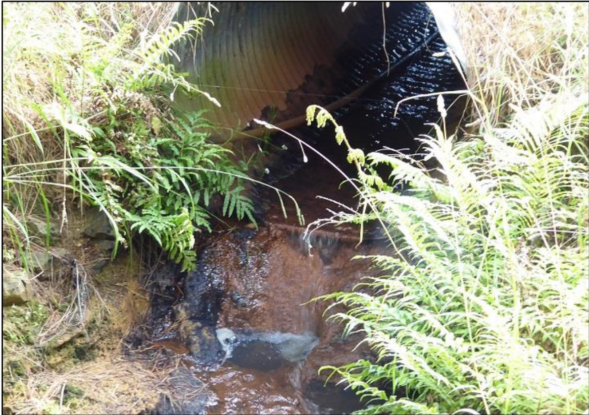
Plate 9 Perched iron culvert on Stream 1 with brown, iron-stained water.
