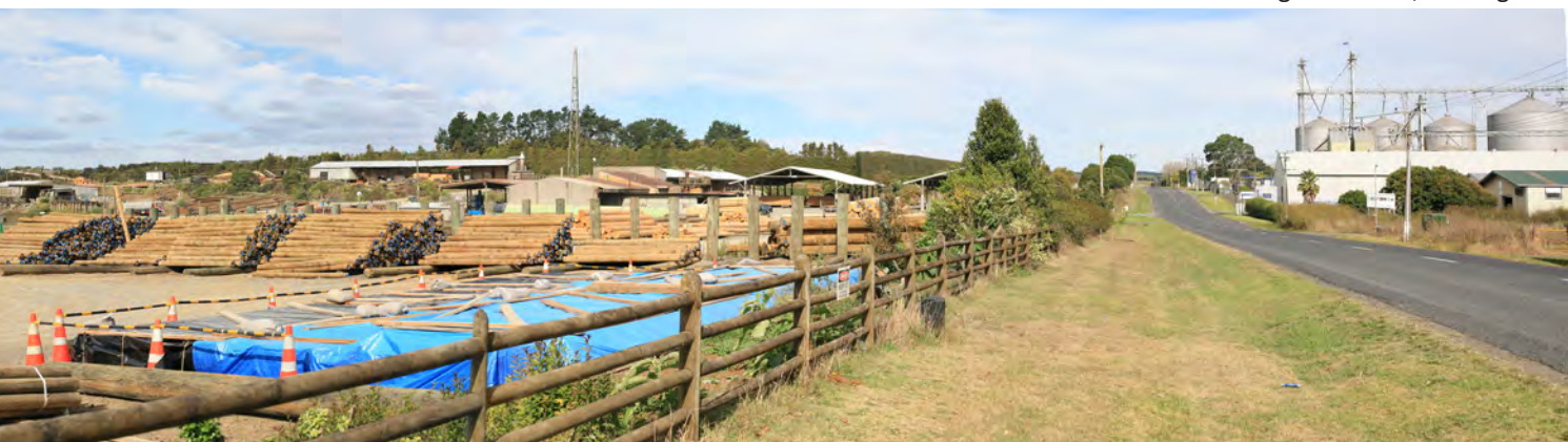
Bollard Road, looking southeast
