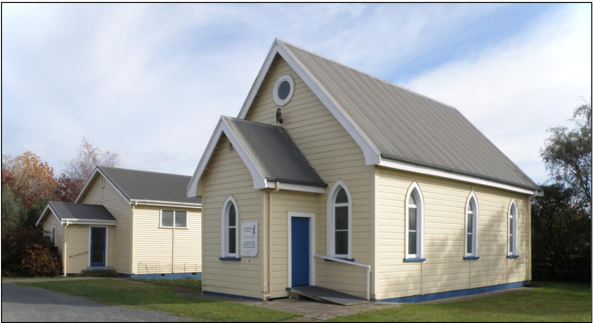
Figure 67 Saint Marks Methodist Church, Te Kowahi (May 2014).
