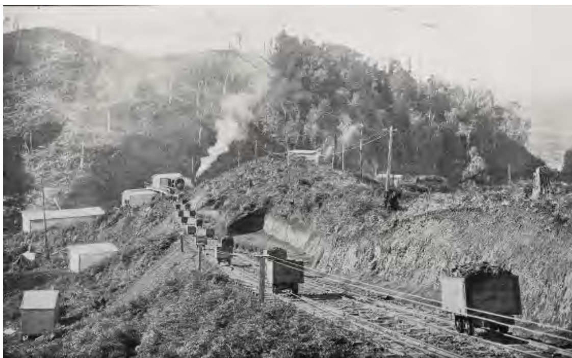
Figure 77: 'Conveying the coal from the mine to the bins: trucks travelling on an endless cable tramway at the Waipa Collieries, near Ngaruawahia'. Auckland Weekly News 30 July 1914, p. 4. AWNS-19140730-45-3, Sir George Grey Special Collections, Auckland Libraries.
