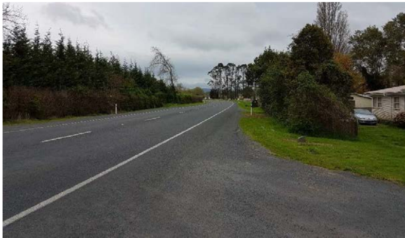
Figure 7: Sight Distance Looking West
