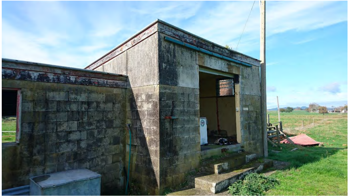
PLATE 13: DETERIORATED SUSPECTED ACM ON ALLOT 405 MILKING SHED
