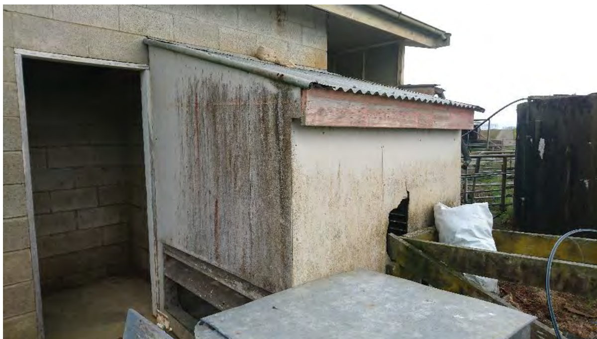
PLATE 8: DAMAGE AND DETERIORATED SUSPECTED ACM ON LOT 2 MILKING SHED
