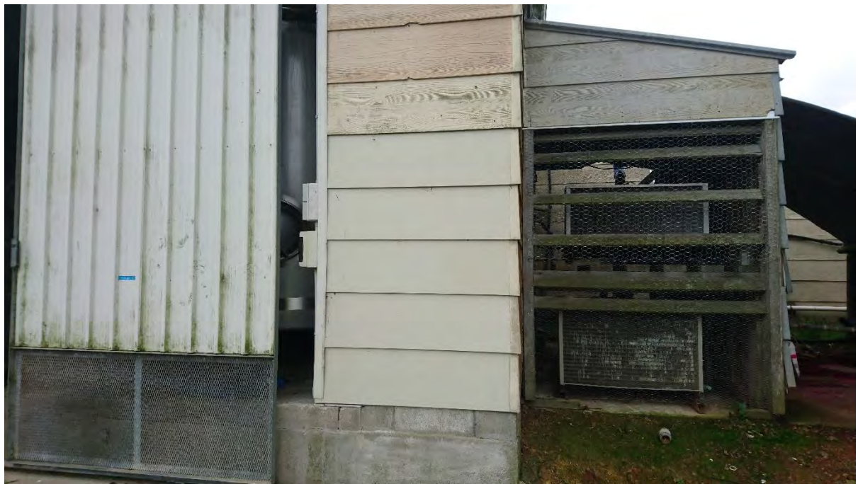
PLATE 5: REPLACED CLADDING PANELS ON LOT 1 MILKING SHED SOURCE OF SUSPECTED ACM FRAGMENTS
