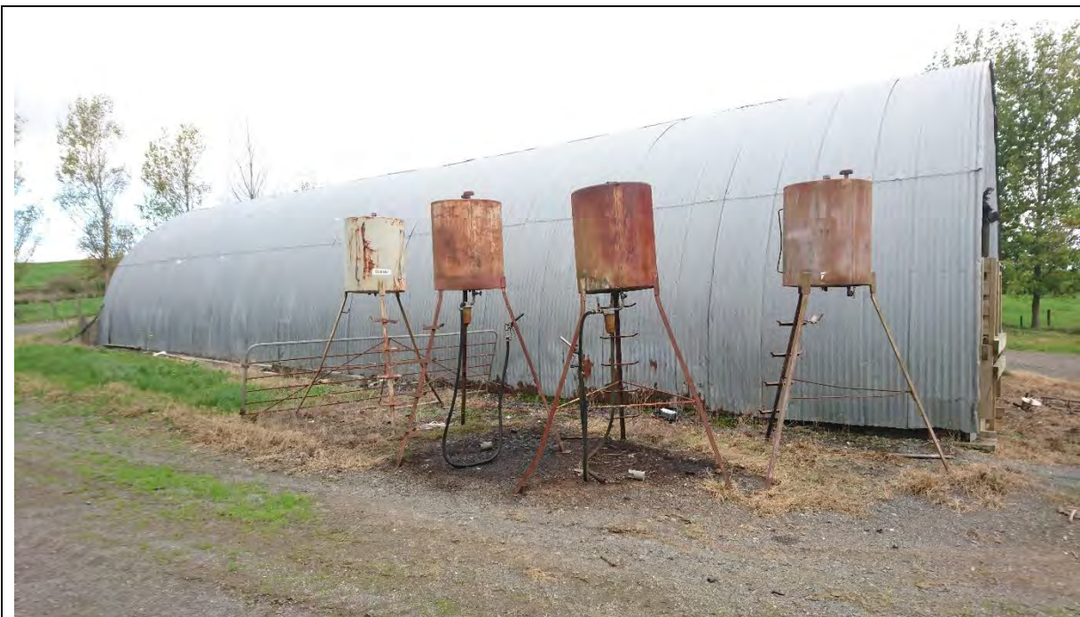
PLATE 3: ABOVE GROUND DIESEL STORAGE TANKS WITH STAINS ON HARDSTAND SURFACE
