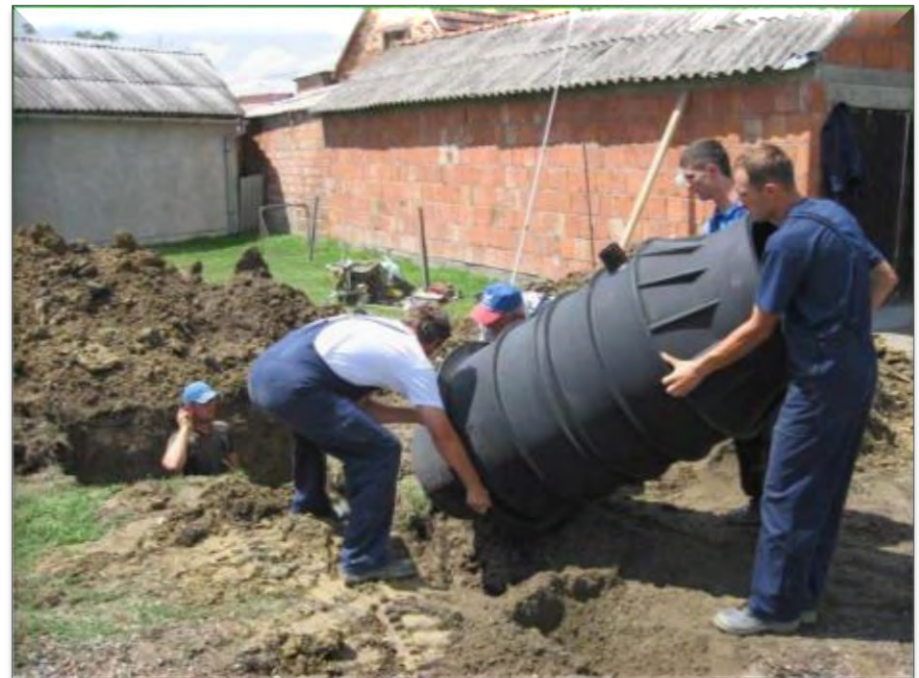
Installing a pre-assembled PE Pit, Rakova Jelsa, Slovenia
