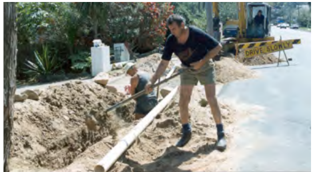
INSTALLATION Shallow trenches ensure low installation costs.
