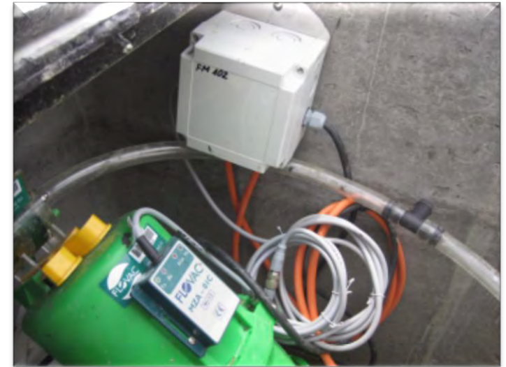
Monitoring the operation of the valve, Zary, Poland
