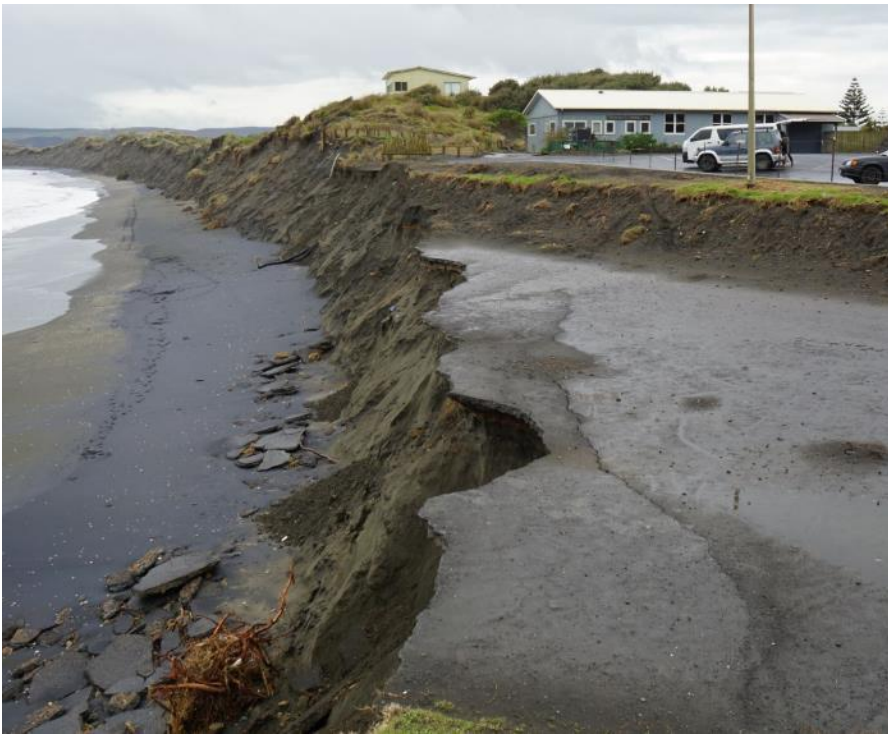
Figure 13: Erosion fronting the car park and private properties at the southern end of Sunset Beach.
