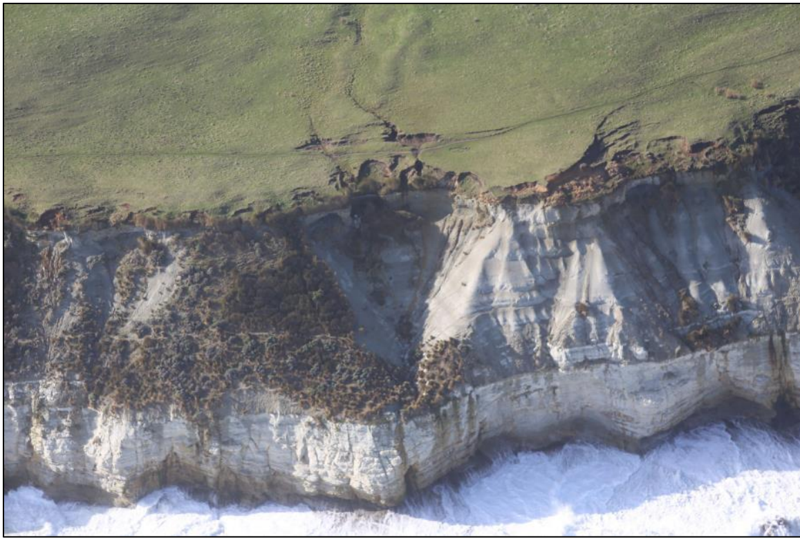
Figure 51: Cliffs between Port Waikato and Raglan (photo Waikato District Council).
