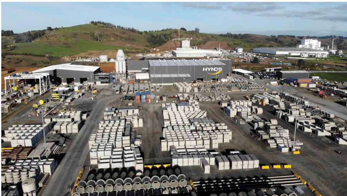
Figure 4. 2020 Image of concrete manufacturing site (east end of McDonald Road site)
