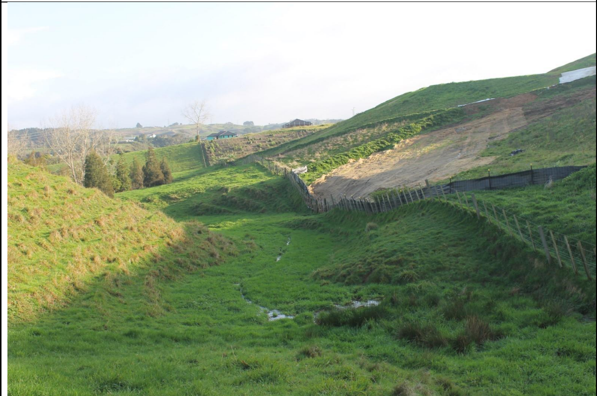
Photo 15. Erosion mitigation middle on Dines Stage 5 property/sub-catchment (looking northwest)
