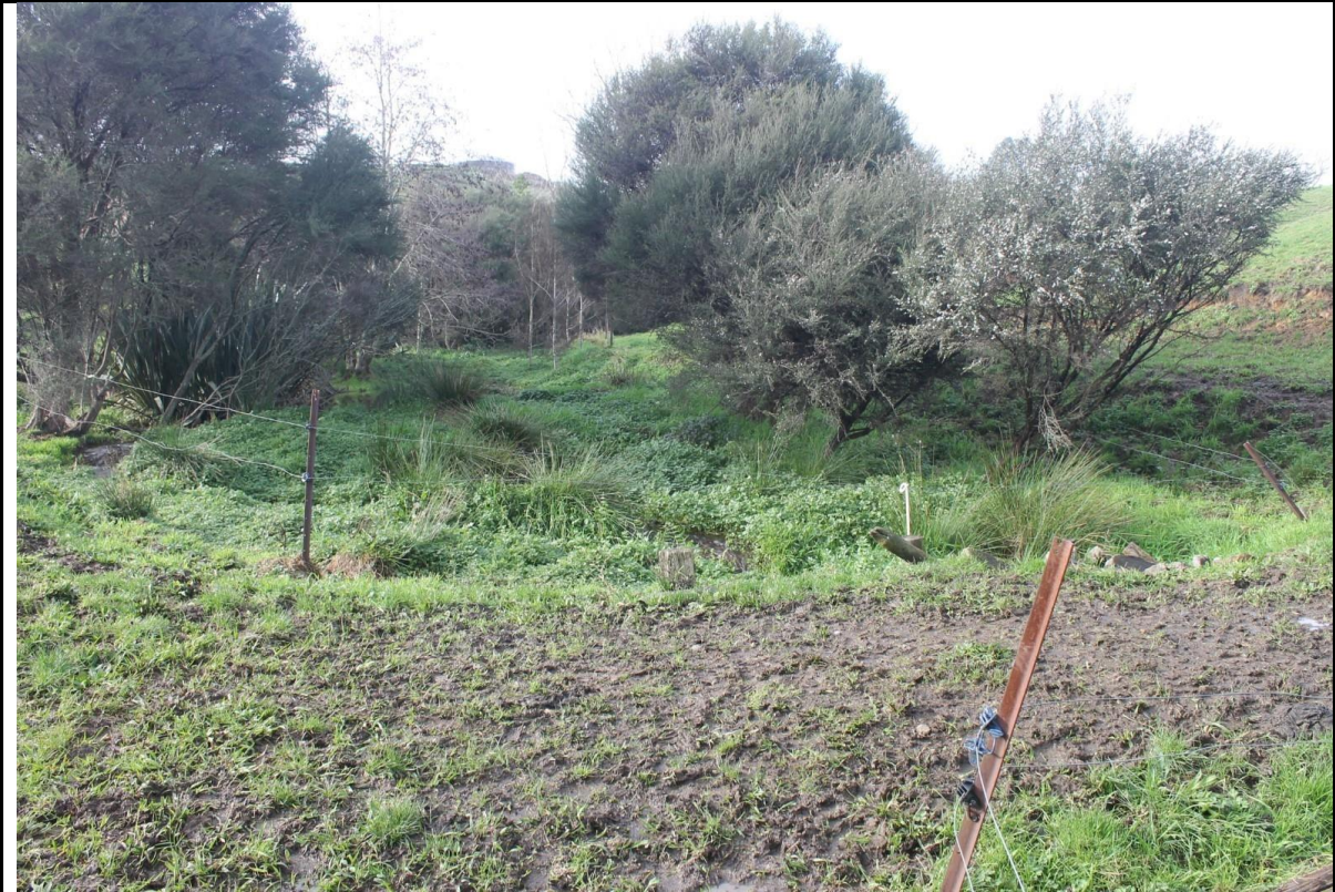
Photo 12. Constructed crossing over main stem stream (looking downstream/west)
