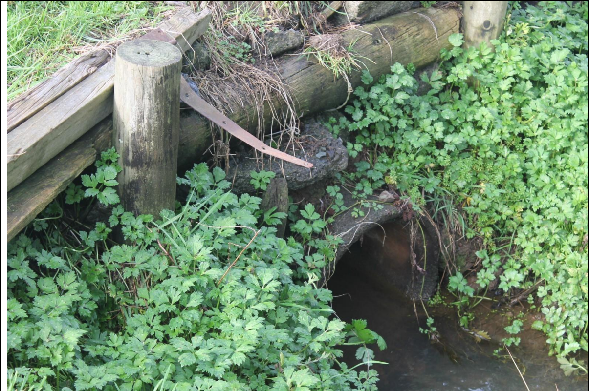
Photo 14. Constructed crossing culvert (looking upstream/east)
