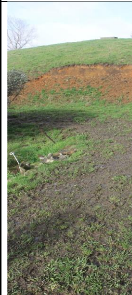
Photo 10. Constructed crossing (looking south)
