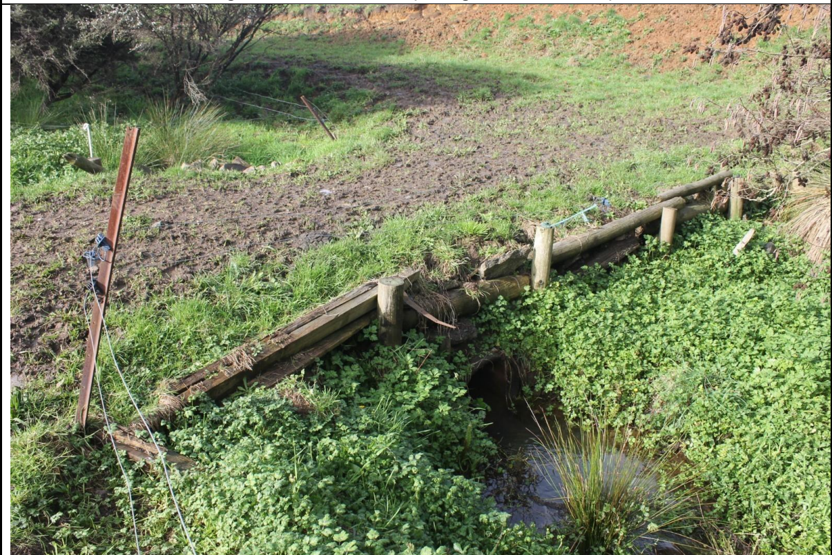
Photo 13. Constructed crossing (looking upstream/east)
