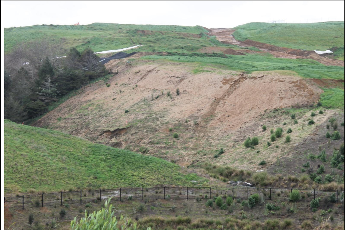
Photo 17. Erosion on Dines Stage 5 property discharging to northern tributary stream upstream of re-routed stream around Wetland D2 that merges with D2 discharge at Noakes Property boundary line (looking northeast)
