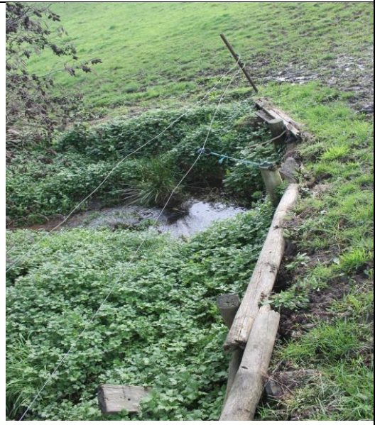
Photo 11. Constructed crossing downstream (looking north)
