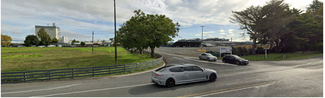
Figure 6: Open Country Dairy and AFFCO buildings set back from Great South Road (Google Maps)
