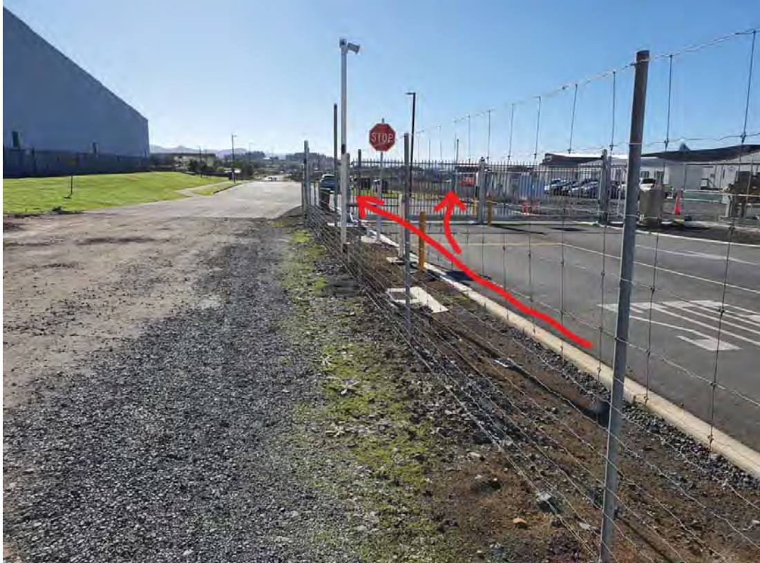
Photo 3 - overland flow would travel in direction of arrows on Synlait site, entering McDonald Road or in events larger than Q100 (or for flows from Synlait land itself), into the ditch on Synlait land.
