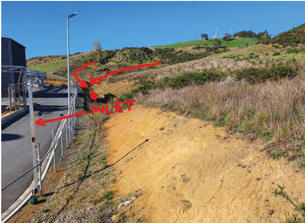
Photo 1 – Looking south. Synlait Channel to inlet piped under Synlait site to ditch in Synlait site parallel to McDonald Road. HVL to the right.
