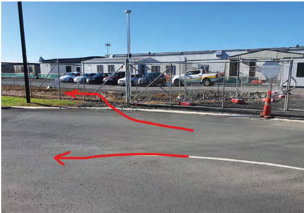
Photo 4 - overland flow would travel in direction of arrows on Synlait site, entering McDonald Road or in events larger than Q100 (or for flows from Synlait land itself), into the ditch on Synlait land.
