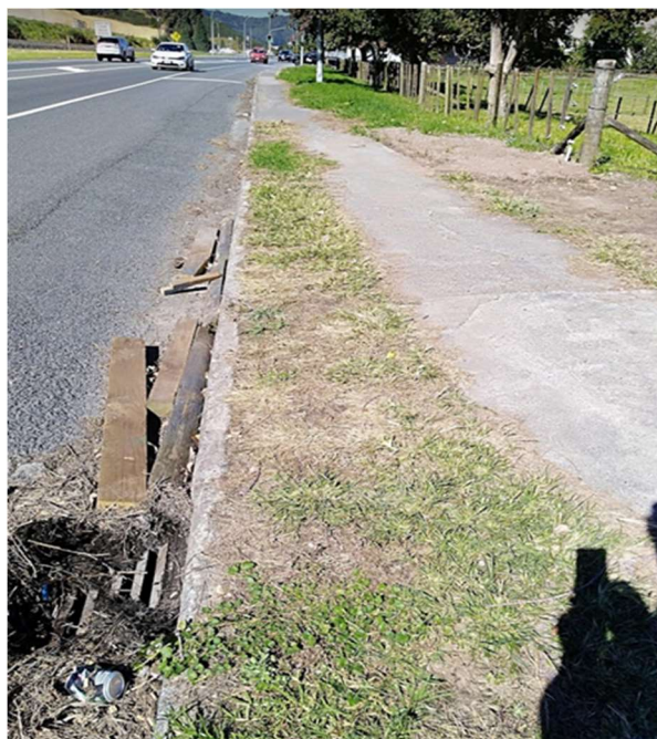
Photo 2: Road catchpit – Proposed Plan Change site right side
