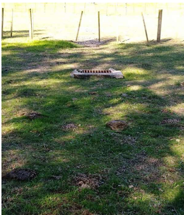
Photo 3: Stormwater Field Grate within Greenfield Area
