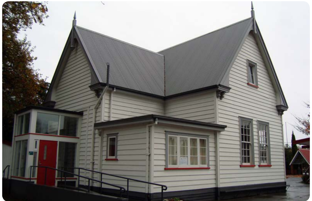
↘ Figure 1. Tamahere School Original Building
