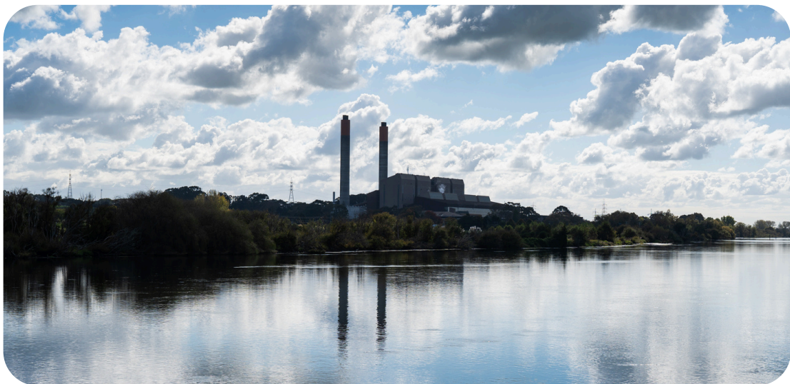
View of Waikato River and the Huntly Power Station
