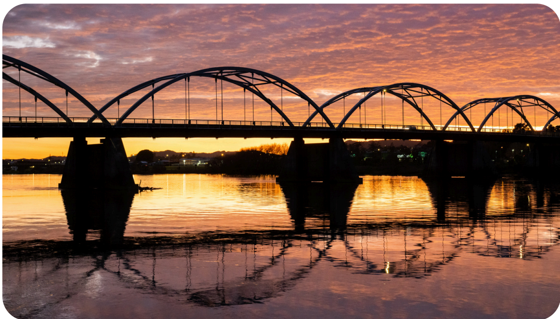
View of Tainui Bridge
