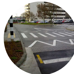
Raised pedestrian crossing
