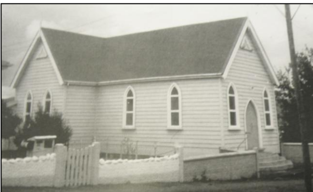
Figure 38 Methodist Church at the site it was moved to in 1974. (Tuakau and Districts Museum Society Inc. n.d. reference #50, Memories , Tuakau Public Library.) 46
