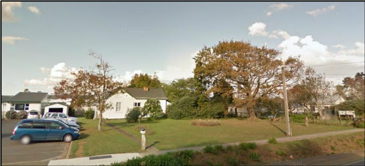
Figure 41 Harrisville School Teachers House, 202 Harrisville Road.
