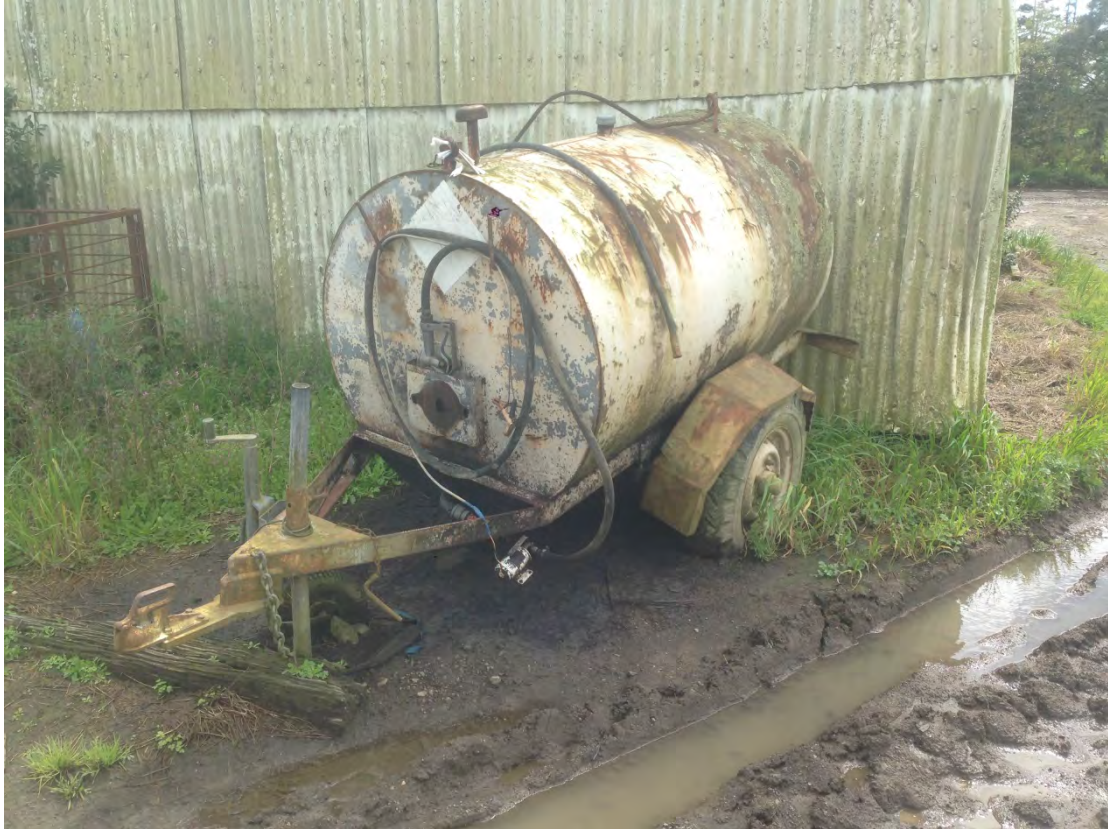
Photograph 1: Photograph looking east showing above ground diesel tank, note staining beneath.
