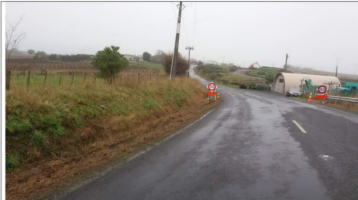
3. Visibility towards the proposed intersection from the north is restricted by the berm height, power poles and vegetation. This is the position of extent of visibility possible within road reserve (requires removal of restrictions/lowering of berm) approximately 110m.
