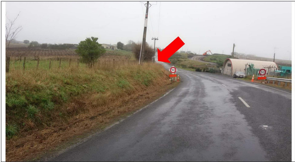
Photograph 3: Approximate position within approaching lane of extent of visibility possible if the berm were lowered and two power poles relocated. (approximately 110m)
