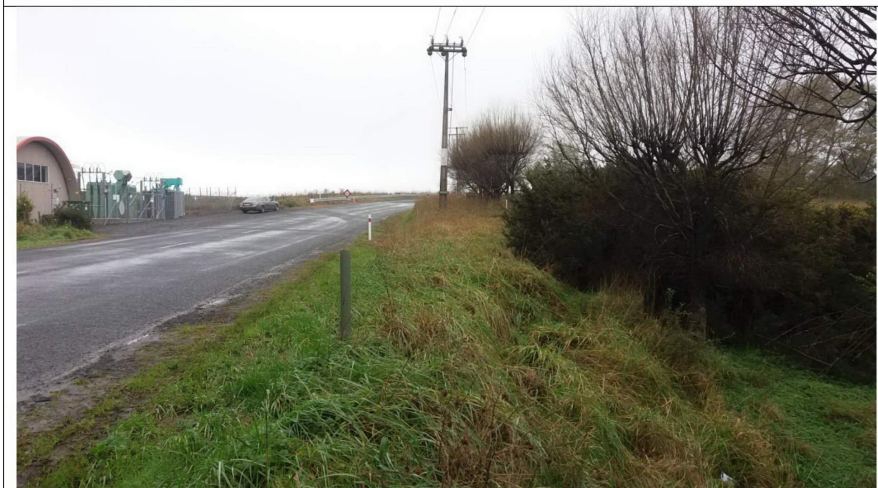
Photograph 2: Existing visibility to the north from the proposed intersection is 90m and is restricted by the bank in the berm, vegetation and power poles.
