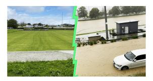
Kāinga Ora and Healthy Waters, lowered the Greenslade Reserve sport fields by a metre and underlaid the turf with a sandy bed to help flood water drain to the harbour.
