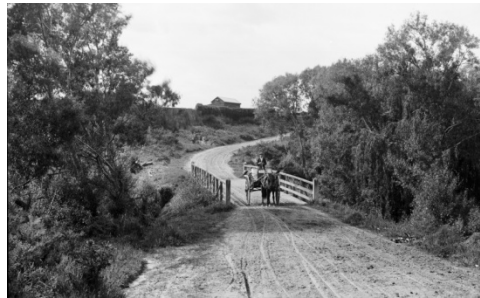
Titled 'On the way to the creamery, Te Kowhai' this shows the County or Main Road in 1909. The first hall is on the rise at rear. The road was formed with clay.
