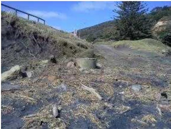
Photograph 12: Site visit in 2014 showing stormwater culvert being covered by further sand.
