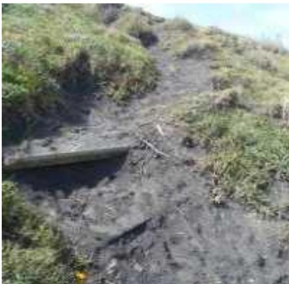
Photograph 14: Concrete telephone poles showing through eroded areas of sand dune below the car park
